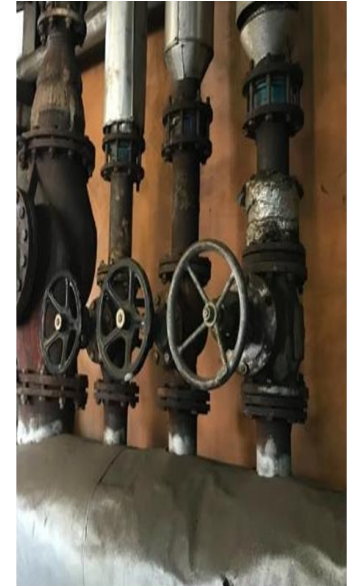
Unlagged Valves contribute to energy loss in steam distribution
