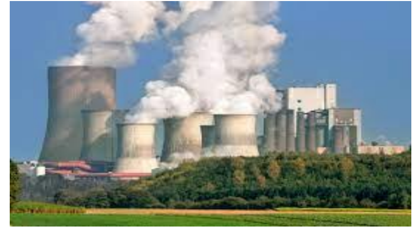
Steam Power Plant
