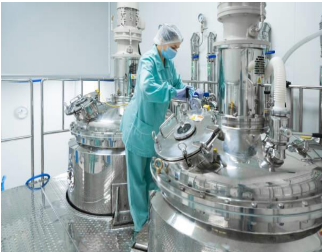
Industrial boiler units installed in a Pharmaceutical plant
